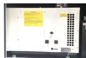
Diesel generator battery charger
