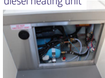
Drying Room diesel heating unit
